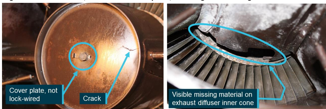
Figure 8: Diffuser area, unsecured cover plate, cracking and missing material
