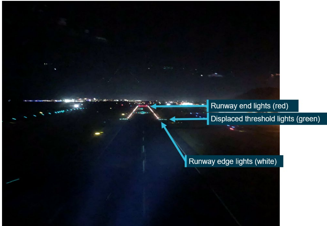
Figure 5: Runway lighting for the runway 15 displaced threshold several nights after the incident
