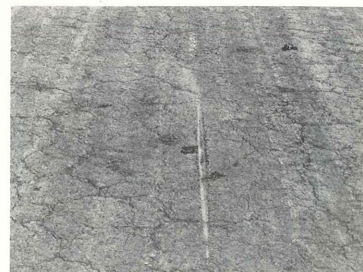
Gouge in strip surface caused by aircraft's tail after power was applied to go around.
