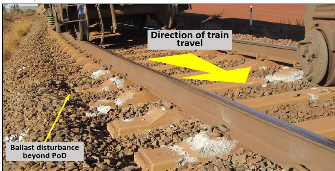
Figure 8: Ballast condition before PoD indicate profile and quality in accordance with Rio Tinto requirements
