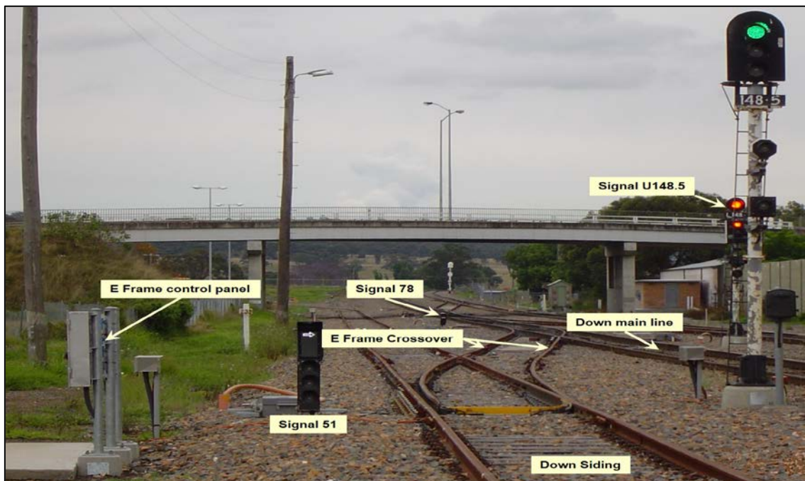
Figure 3: Location E Frame control panel
