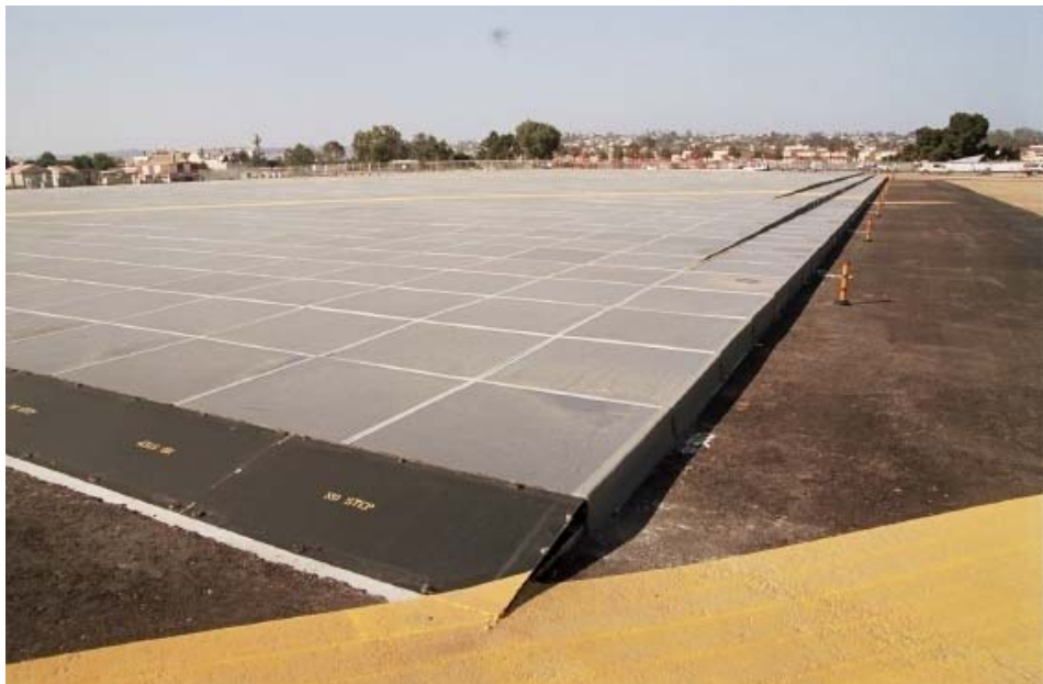
Figure 14: An EMAS transition ramp at San Diego International Airport (KSAN), runway 09 end
