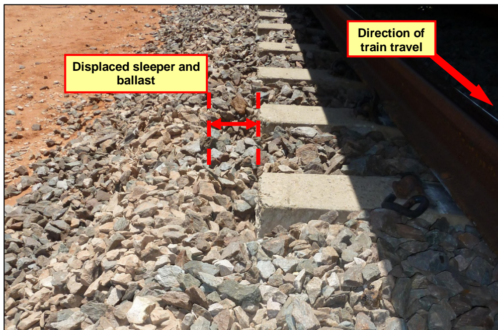
Figure 8: Photograph on northern side of mainline near the POD, shows evidence of horizontal sleeper displacement
