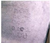
Figs. 24 & 25 Blade repair codes present on the upper surface of the flange.
