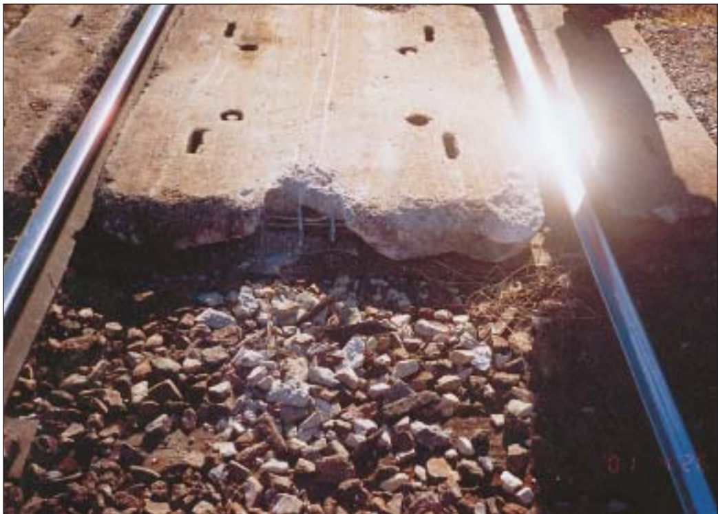
FIGURE 11: Pedestrian crossing showing impact damage to concrete slab in track four foot
