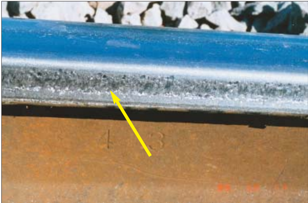
FIGURE 22: High rail gauge face showing wear from lack of lubrication
