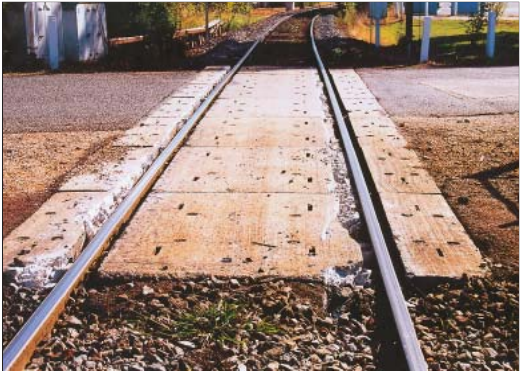
FIGURE 10: Station entry level crossing showing damage to roadway
