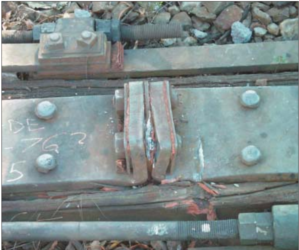
FIGURE 12: Damage to interlocking equipment on a turnout
