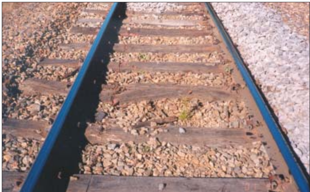
FIGURE 9: Section of track showing damaged sleepers
