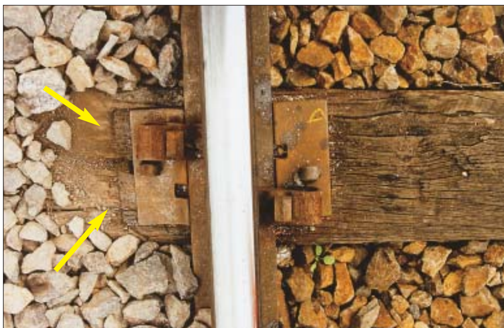
FIGURE 18: TrakLok fastener on high rail showing sleeper wear as a result of plate movement
