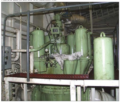
FIGURE 2: Lube oil Boll and Kirch automatic filter
