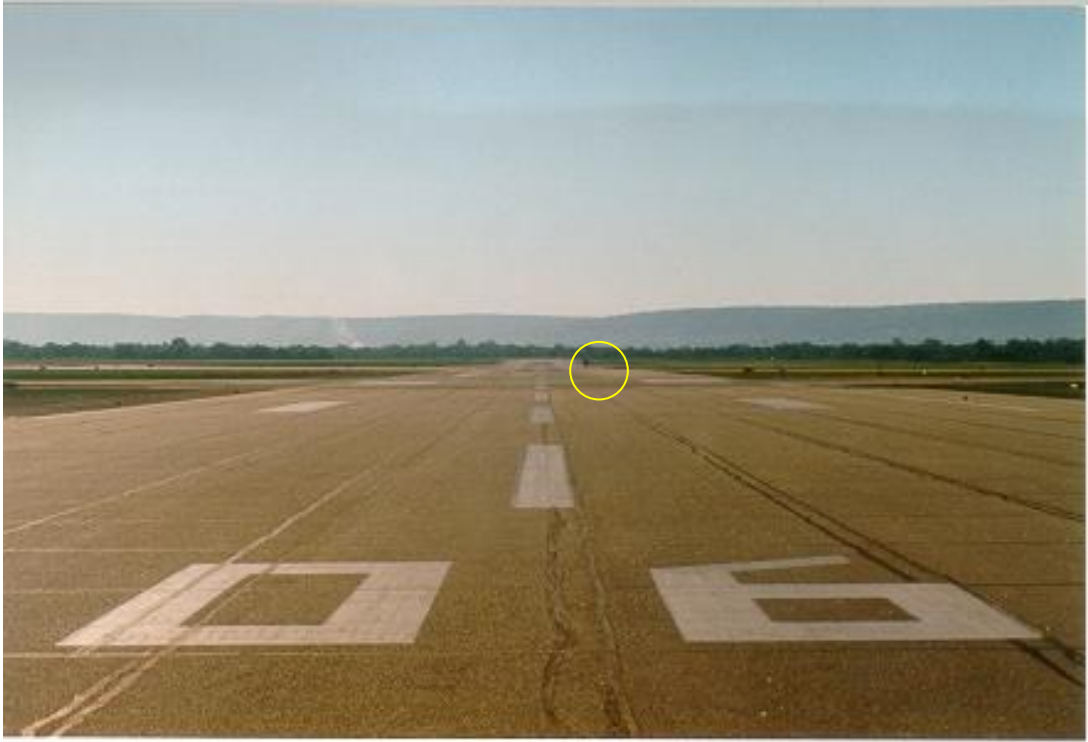
FIGURE 6: View from aircraft of sweeper from runway 06 threshold
