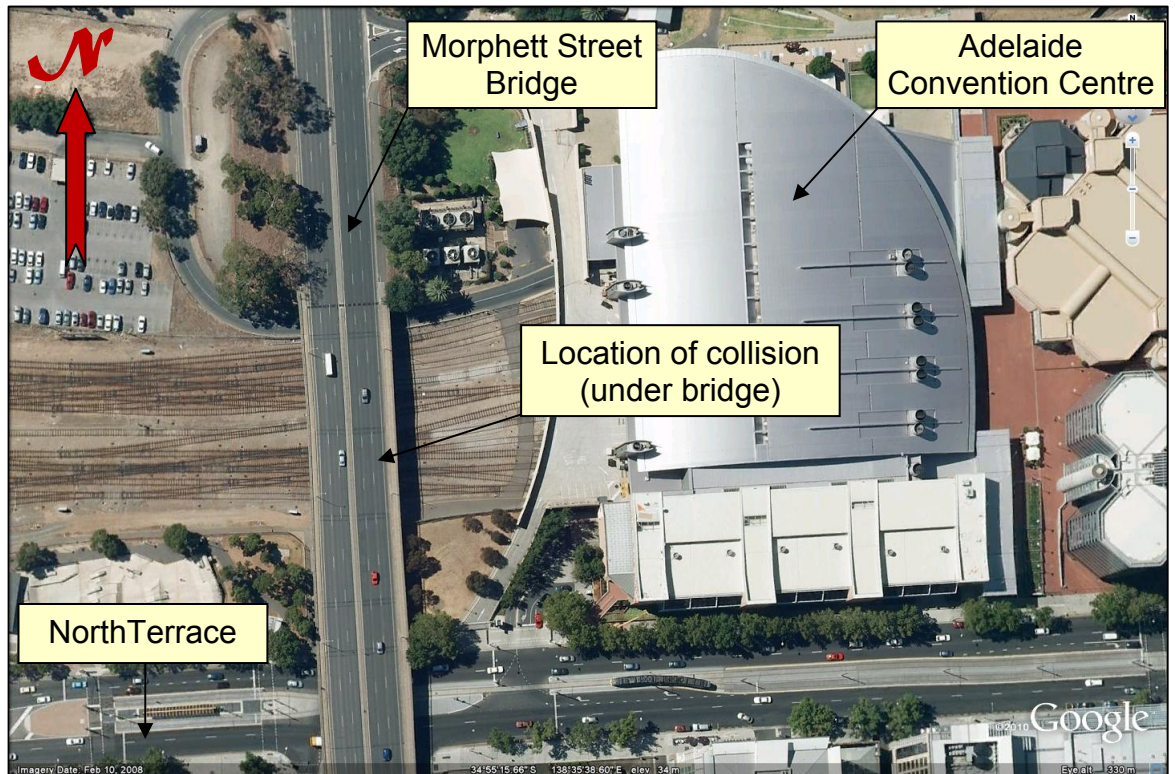
Figure 2: Aerial view – Adelaide Railway Station, South Australia
