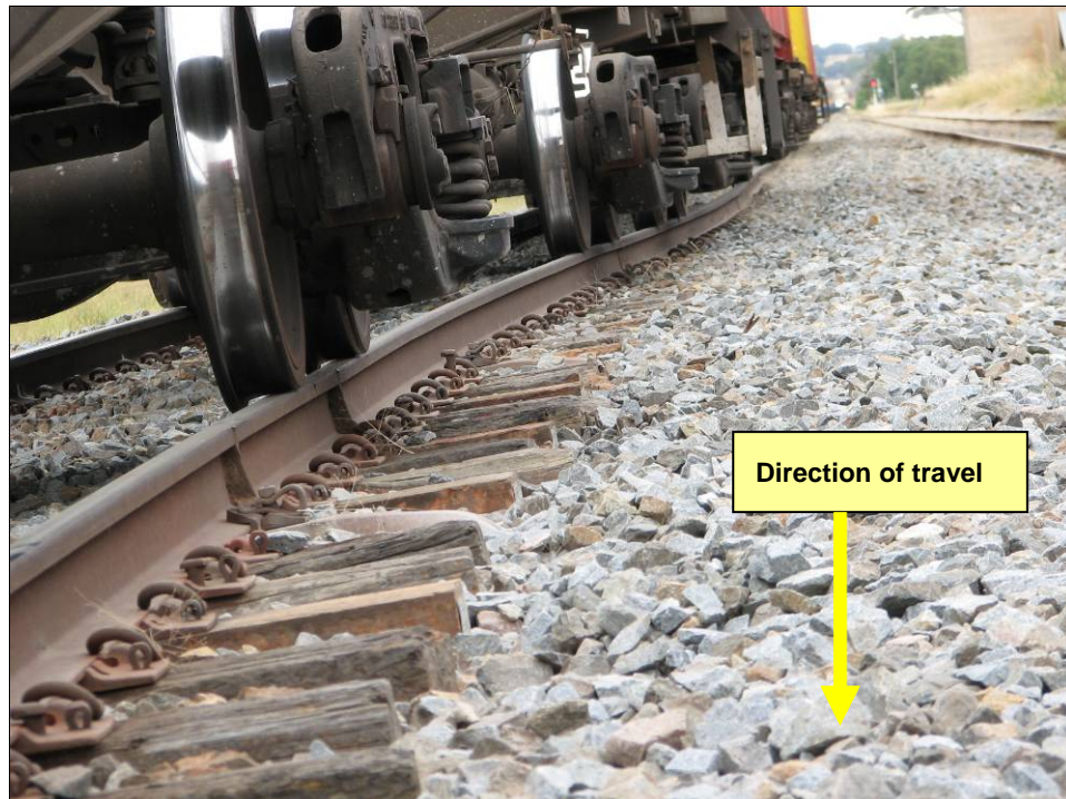
Figure 12: Misaligned track under last wagon of the derailed portion RRY 23
