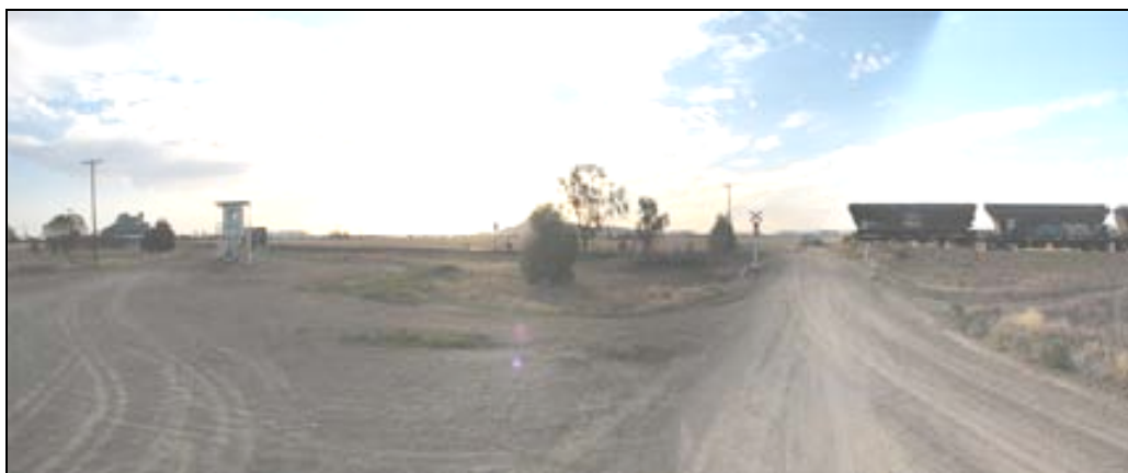
Figure: 12 Photograph of the approach to the level crossing
