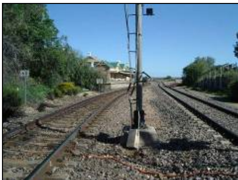
Figure 4: Photographs of damage to signal 23 at Murray Bridge
