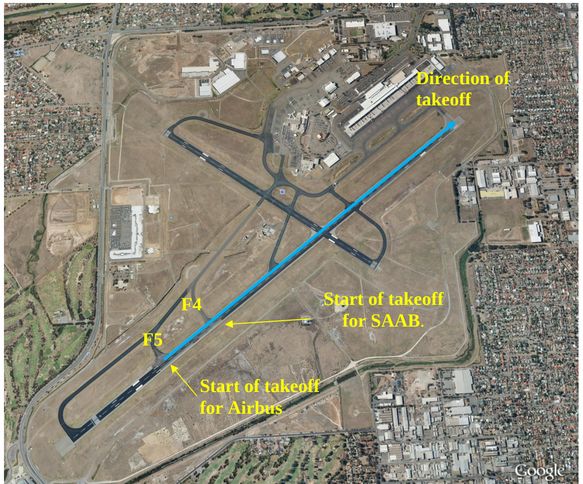
Figure 1: Adelaide Airport showing positions of taxiways F4 and F5 (Google Earth)
