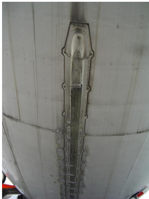
Figure 1: Damaged tail strike indicator and skin
