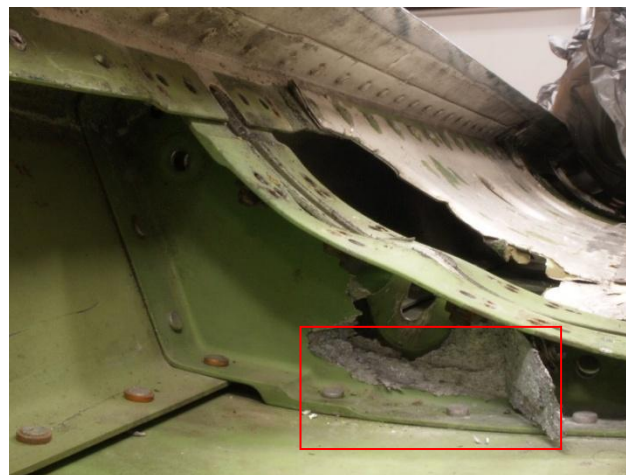
Figure 5: Outboard auxiliary track attachment corrosion
