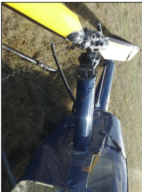
Figure 6: Instructor's headset cable and main rotor mast
