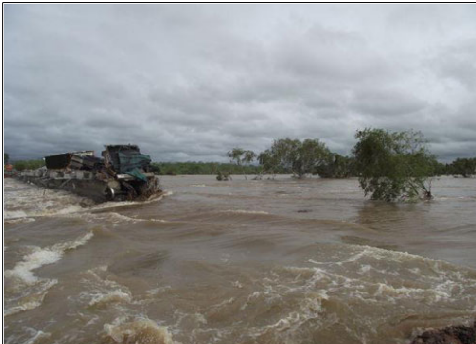
Figure 13: South-eastern approach to Edith River rail bridge about 1 hour after the derailment
