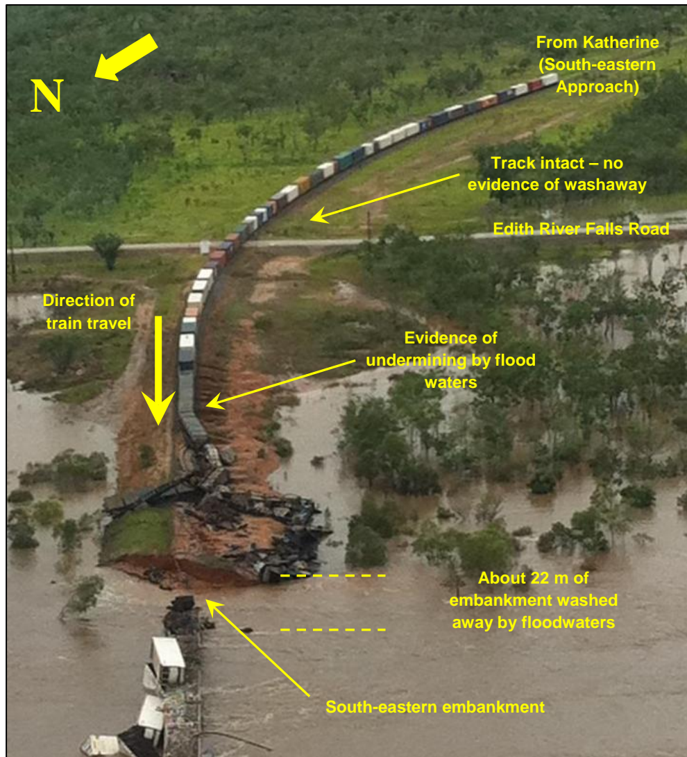
Figure 10: Approach to Edith River rail bridge early on 27 December 2011
