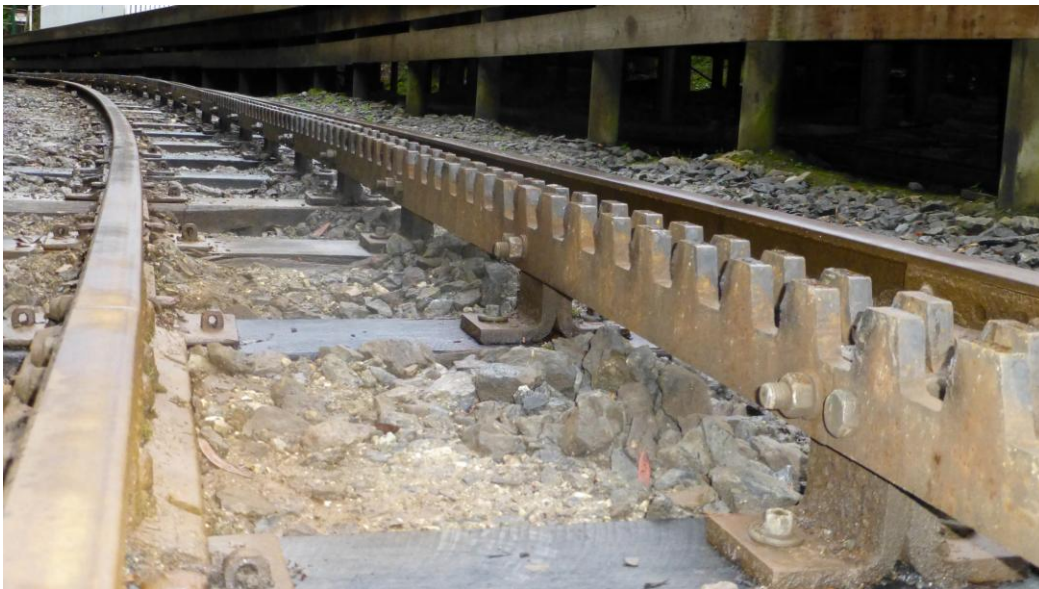
Figure 5: The Abt rack
