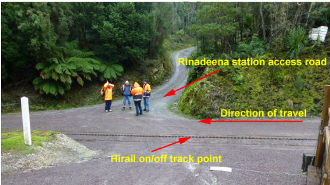
Figure 3: Rinadeena Station access road and vehicle on/off point
