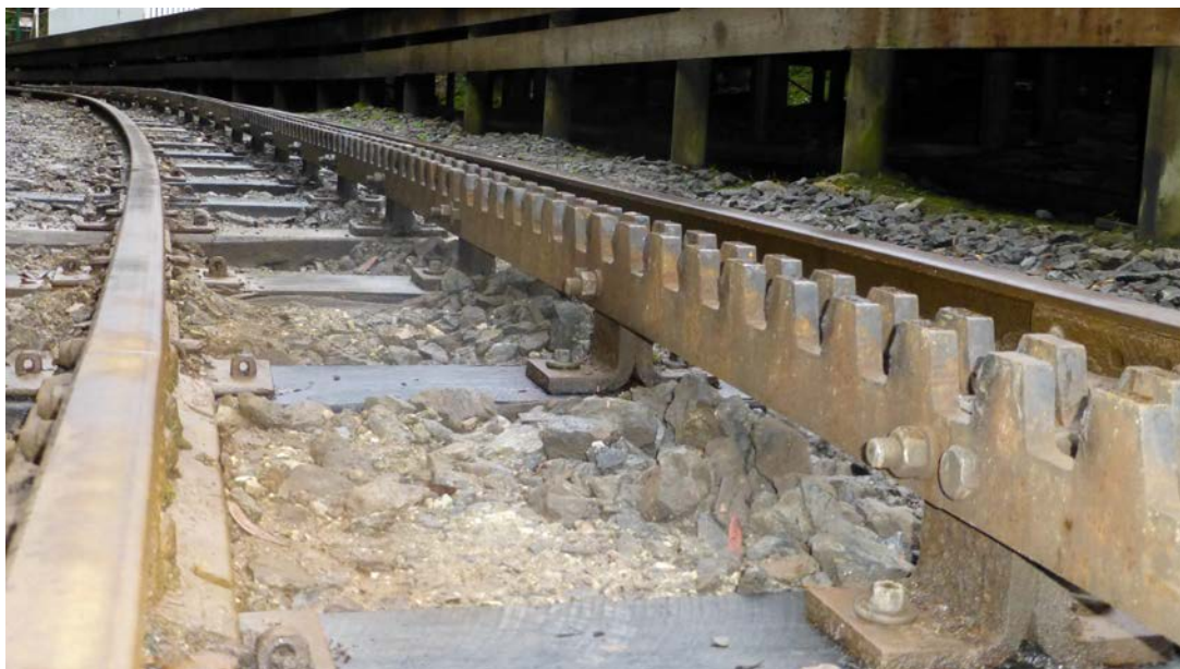
Figure 5: The Abt rack
