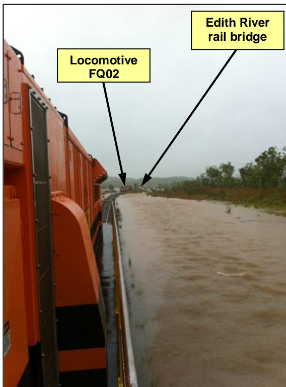
Figure 5: View from lead locomotive GWA001, looking south towards Edith River, about one hour after the derailment.
