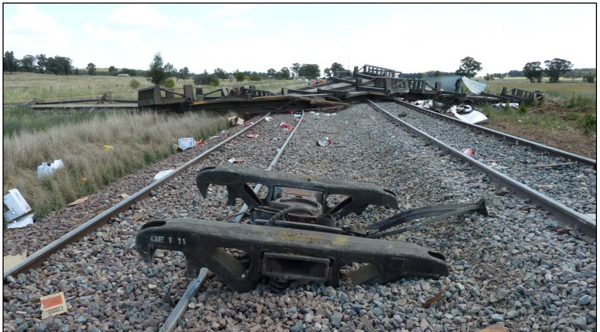
Figure 1: Last four wagons of train 7SP5 at the Wurrinya derailment site
