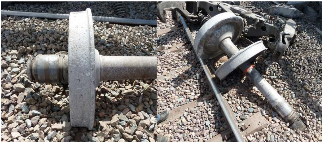
Figure 6: Wheels from southern end of Wirrinya with damage indicative of having run derailed for some distance
