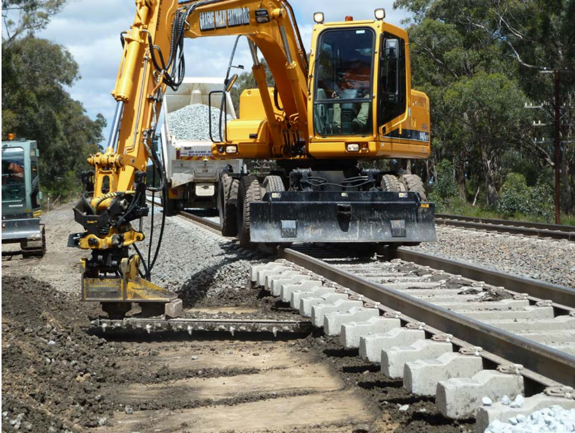
Figure 36: Remediation work – track under-cutting
