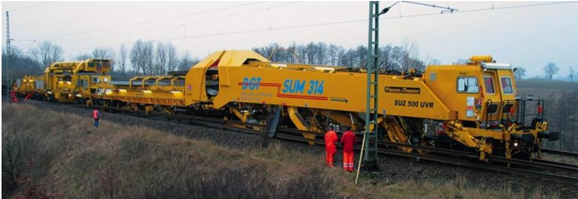
Figure 22: Plasser SUZ 500 UVR Track Relaying Machine
