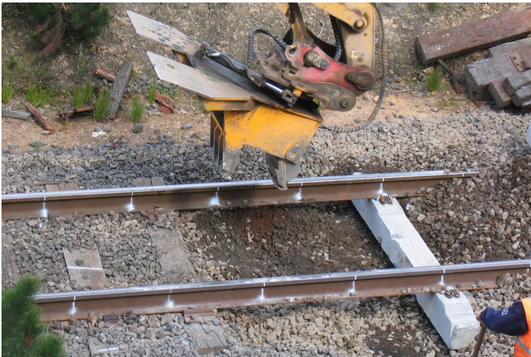
Figure 26: Concrete sleeper clipped in position
