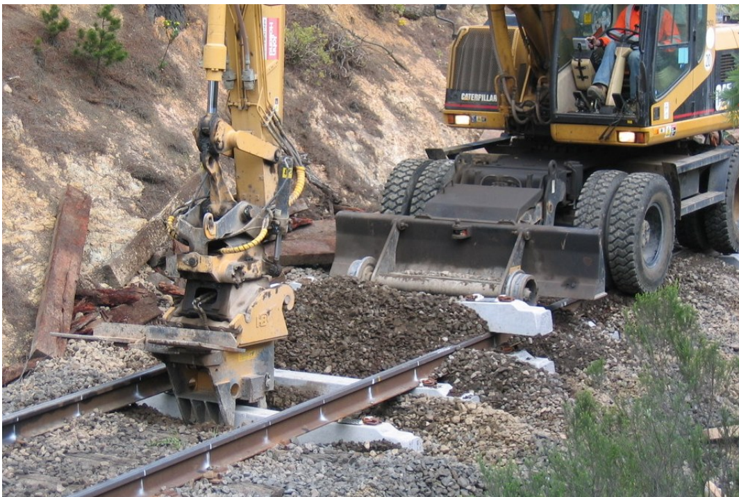
Figure 25: Inserting a concrete sleeper using a Platypus attachment
