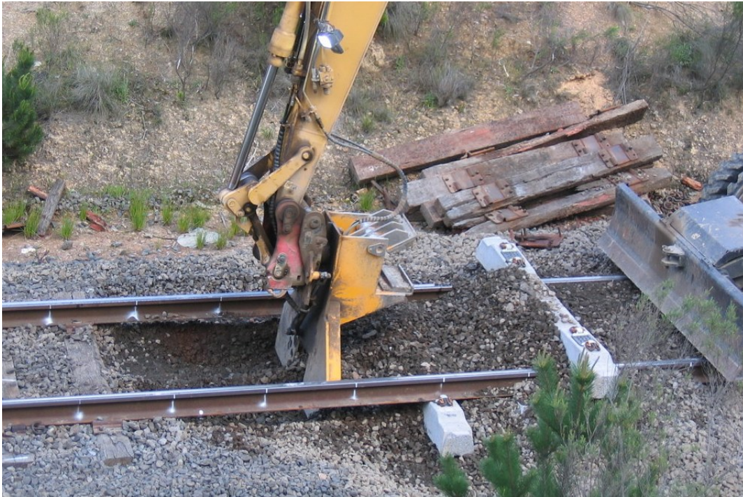
Figure 24: Scarifying the ballast with a Platypus attachment
