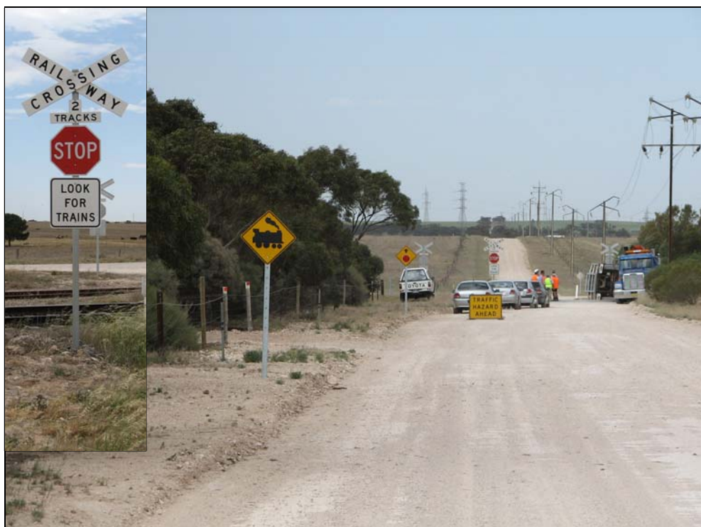
Figure 3: Stop and approach warning signs (Inset 'Stop' sign assembly) approaching the level crossing.
