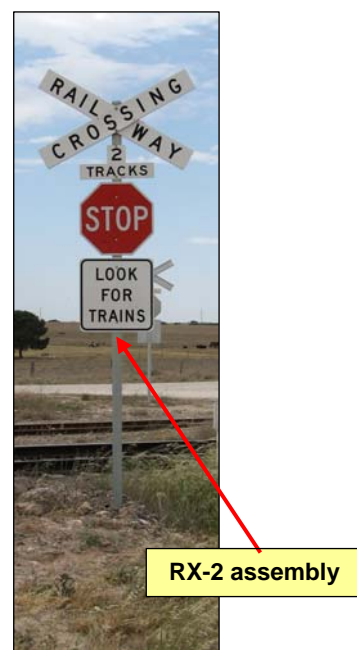
Figure 13: Left photograph of advance warning sign W7-7(L), W3-1 and 'Stop' sign assembly RX-2, right photograph RX-2 assembly.
