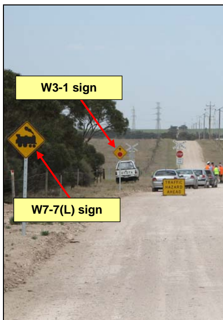
Figure 13: Left photograph of advance warning sign W7-7(L), W3-1 and 'Stop' sign assembly RX-2, right photograph RX-2 assembly.
