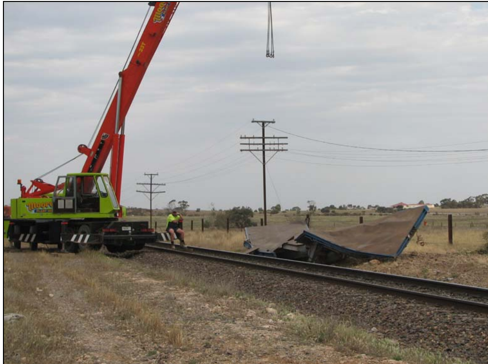
Figure 8: Photo of site recovery, damaged trailer approximately 85 m from collision site.
