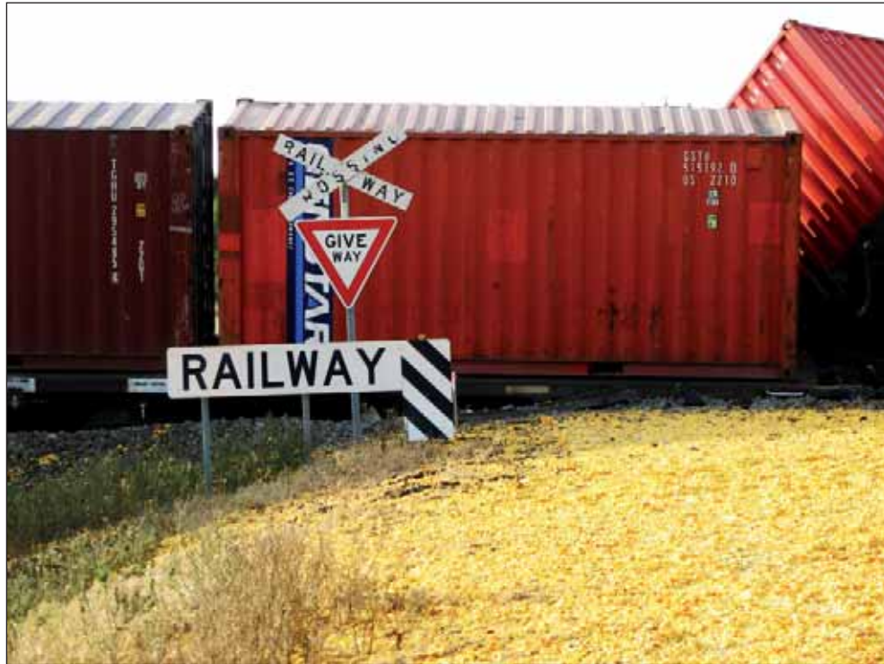
Figure 2: Give way assembly and left side railway level crossing width marker assembly located on the southern approach to the level crossing (northern side destroyed)
