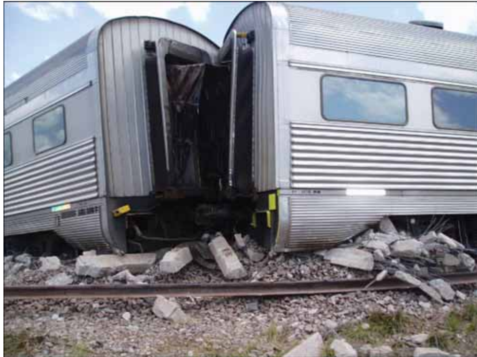
Figure 28: Vestibule area between connected carriages
