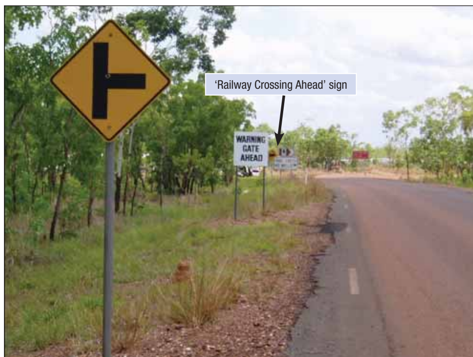
Figure 34: Sign Clutter - Fountain Head Road level crossing, Ban Ban Springs (southern approach)
