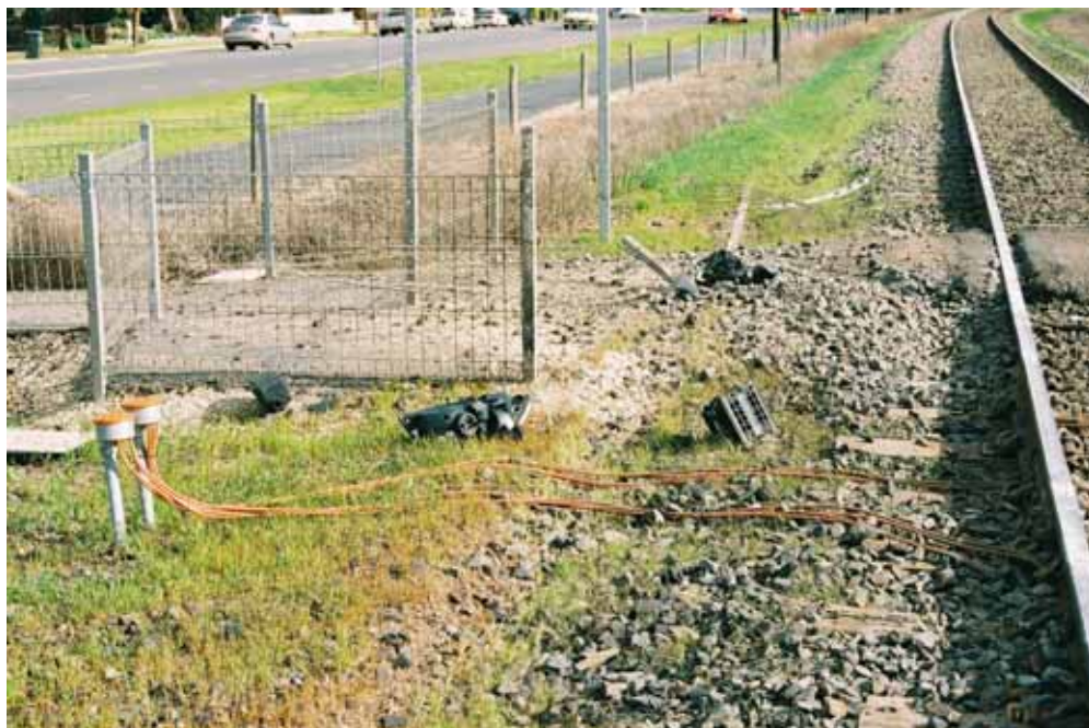
Figure 4: Damage caused by the motor vehicle colliding with the near-by pedestrian crossing. (Photograph, courtesy of Victoria Police).
