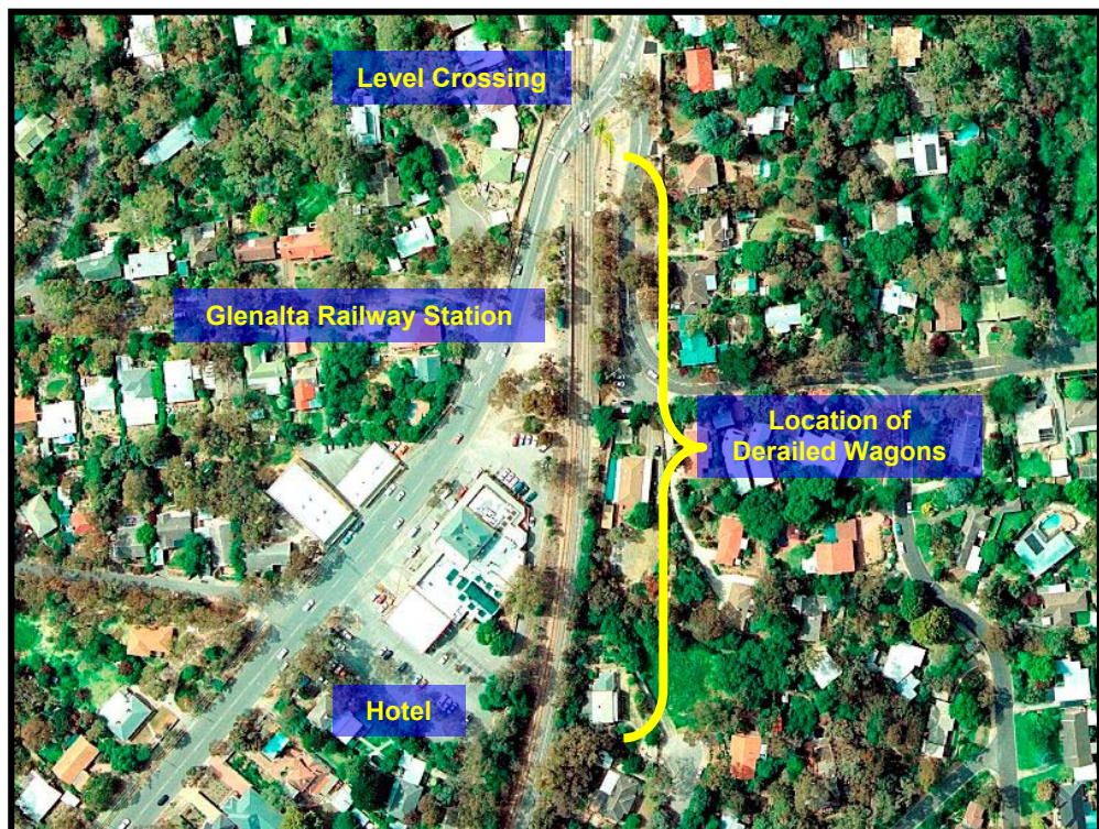
Figure 3: Aerial photograph of Glenalta, South Australia
