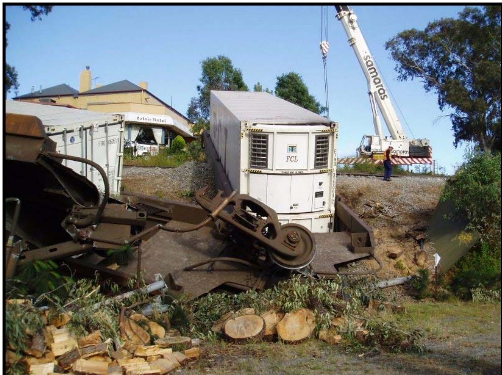
Figure 20: View of rollingstock in private property and recovery process
