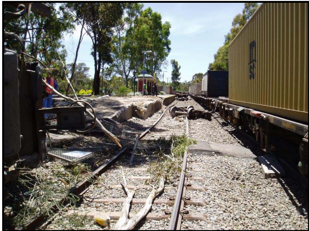
Figure 1: View of TransAdelaide track and Glenalta Railway Station platform
