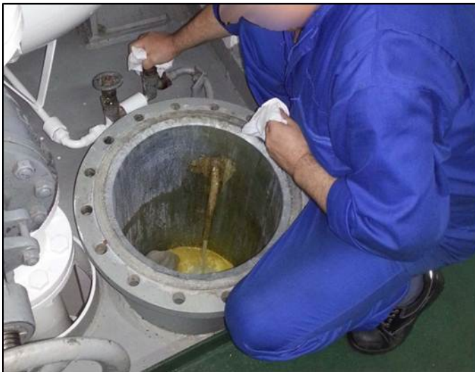
Figure 5: Draining condensate from number one main air receiver, after the accident
