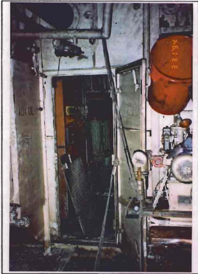
Forward bulkhead door, showing six securing dogs
