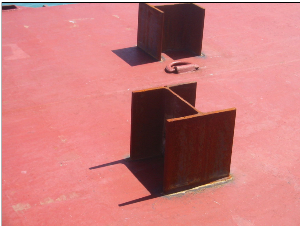
Figure 2: Stoppers welded to the hatch covers.
