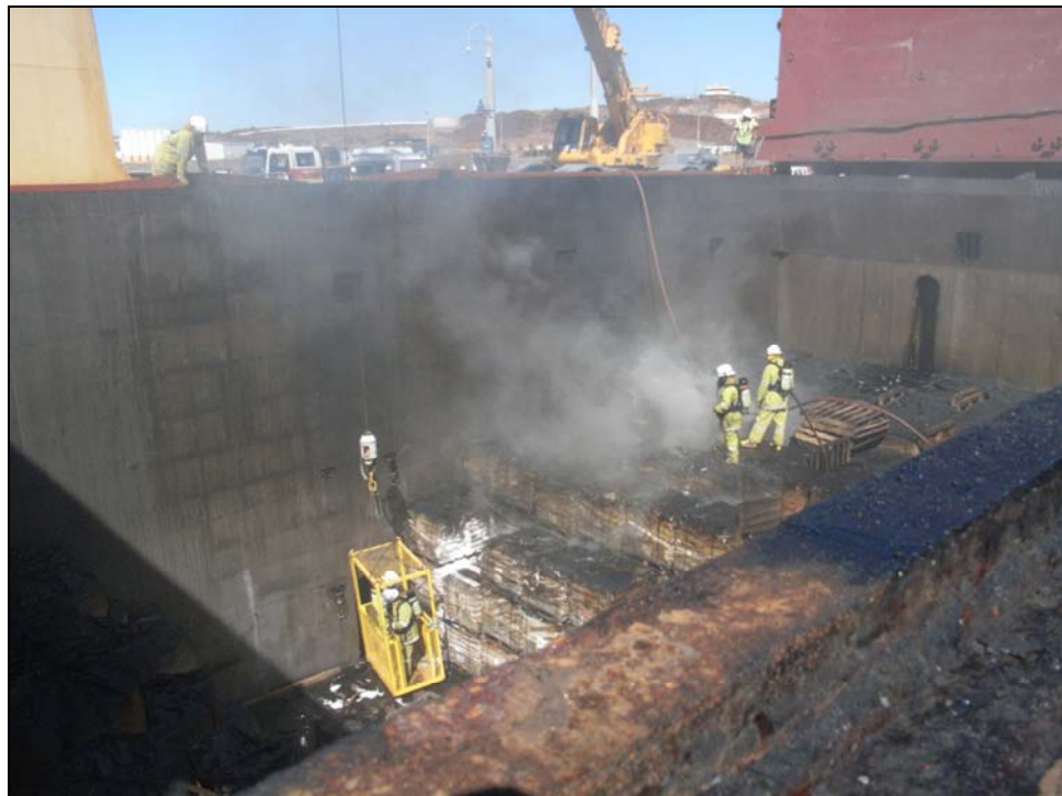
Figure 4: Fire fighters attempting to access the seat of the fire
