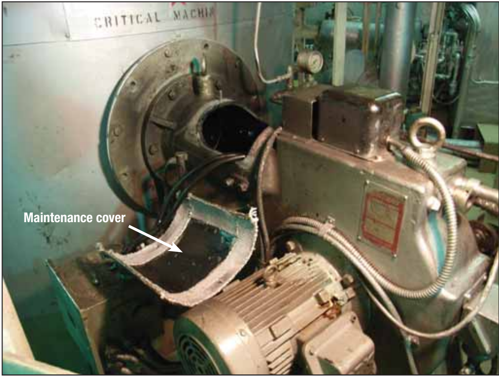
Figure 4: Volcano VJ-140-1 oil firing unit
