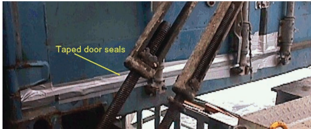
Figure 4: Taped door seals of the container in Figure 3
