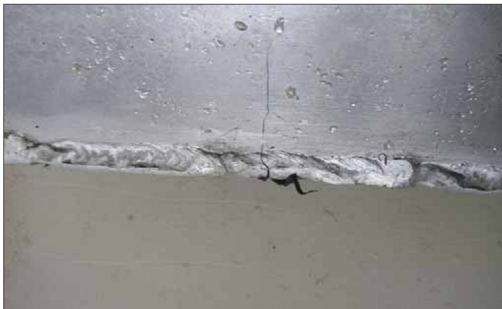
Figure 23: Fuel tank weld quality
