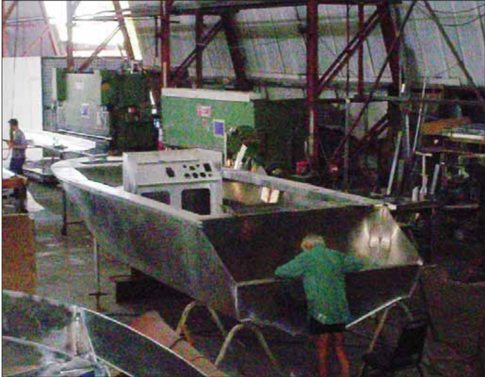
Figure 8: The IRVs under construction at Subsee
