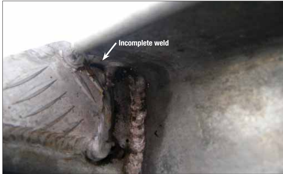
Figure 14: Leak in Zueber Erkep's cockpit deck
