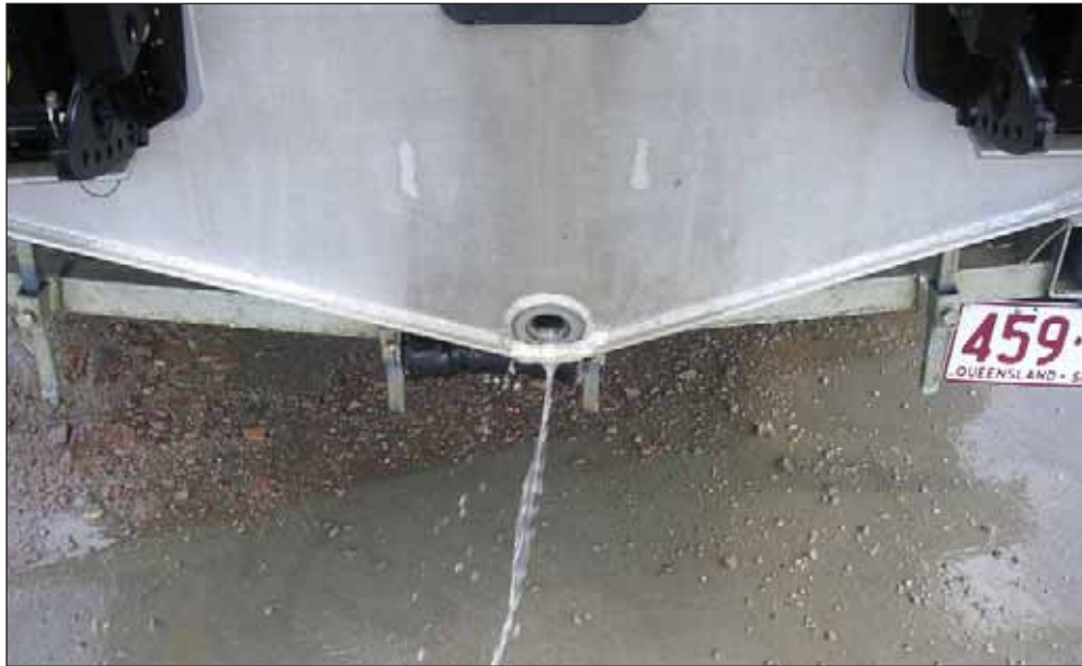
Figure 15: Water being drained from the under deck void space
