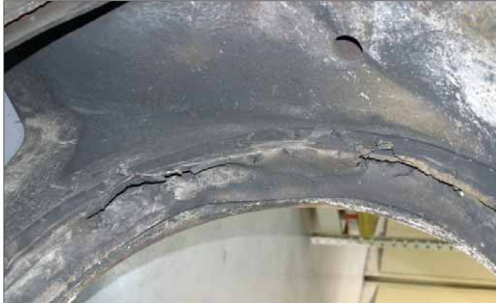
Figure 4: Remanents of the turbine shroud assembly
