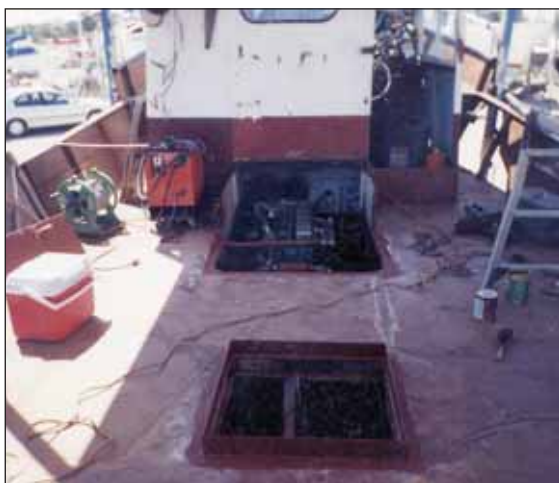
FIGURE 2: Modification work proceeding on Tamara's hatches
