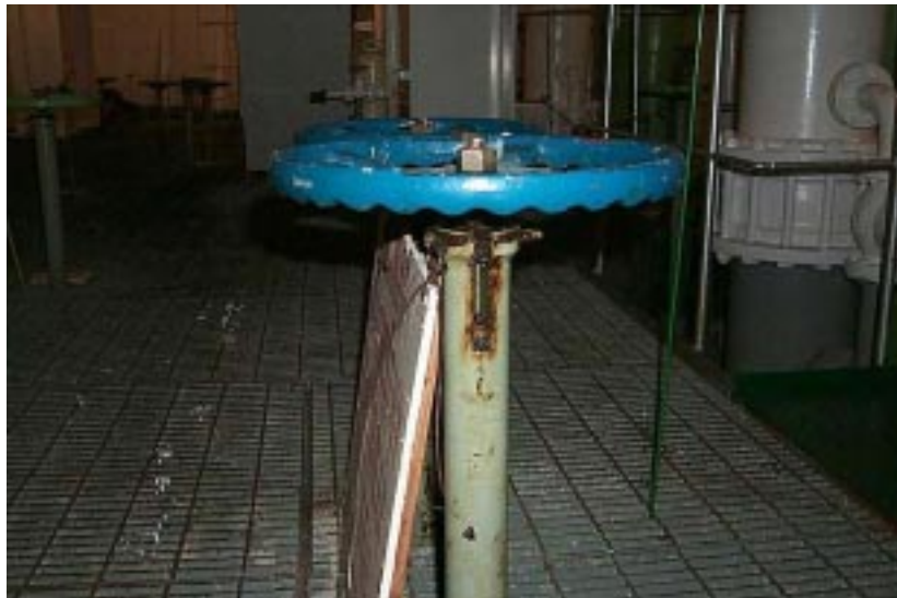
Figure 5 Sea-chest valve spindles showing position indicator
