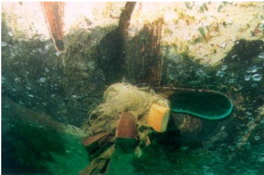
FIGURE 9 Repair with wooden plugs and Denso tape
