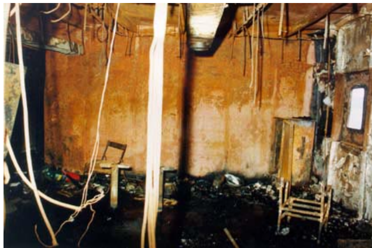
Showing portside of 1st Engineer's day room.
