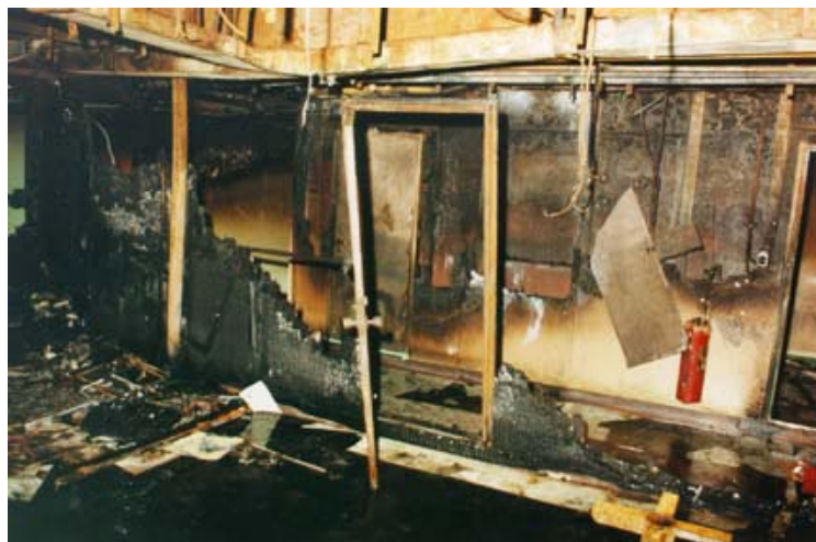
Doorway and remains of bulkhead between 1st Engineer's cabin and cross-alleyway
