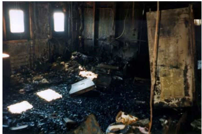
Master's cabin looking forward and to starboard
