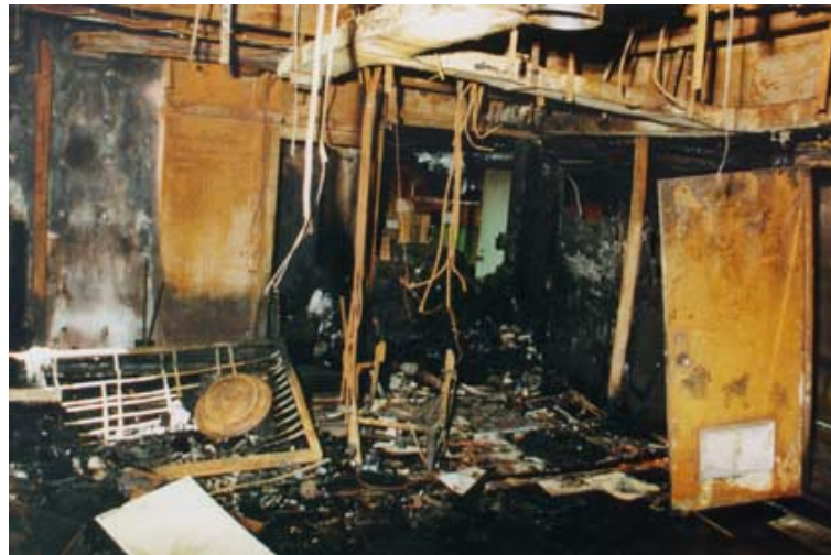
Interior of 1st Engineer's cabin, from day room into bedroom, remains of bed bottom left
