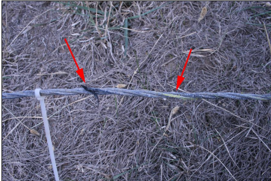
Figure 3: Black and yellow markings observed on the severed conductor, indicative of contact with the spray hoses and fittings
