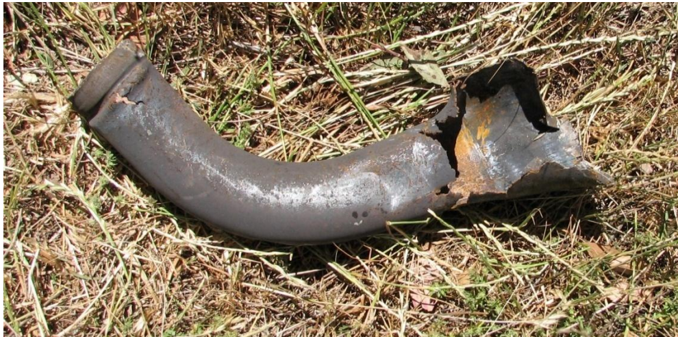
Figure 9: Fractured exhaust pipe as found on site
