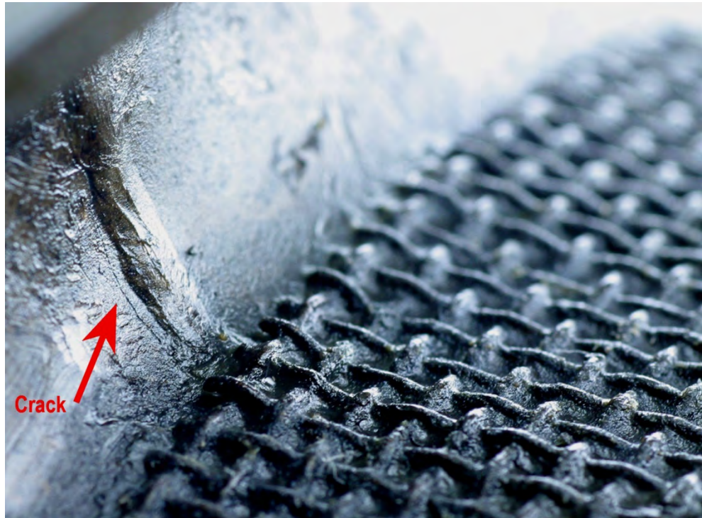
Figure A10: Close view of the right-side ‘armpit’ crack, as shown in Figure A5
