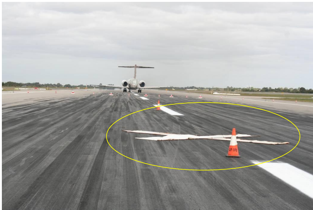
Figure 1: Runway 21 works area looking south. Note the 6m cross (circled)
