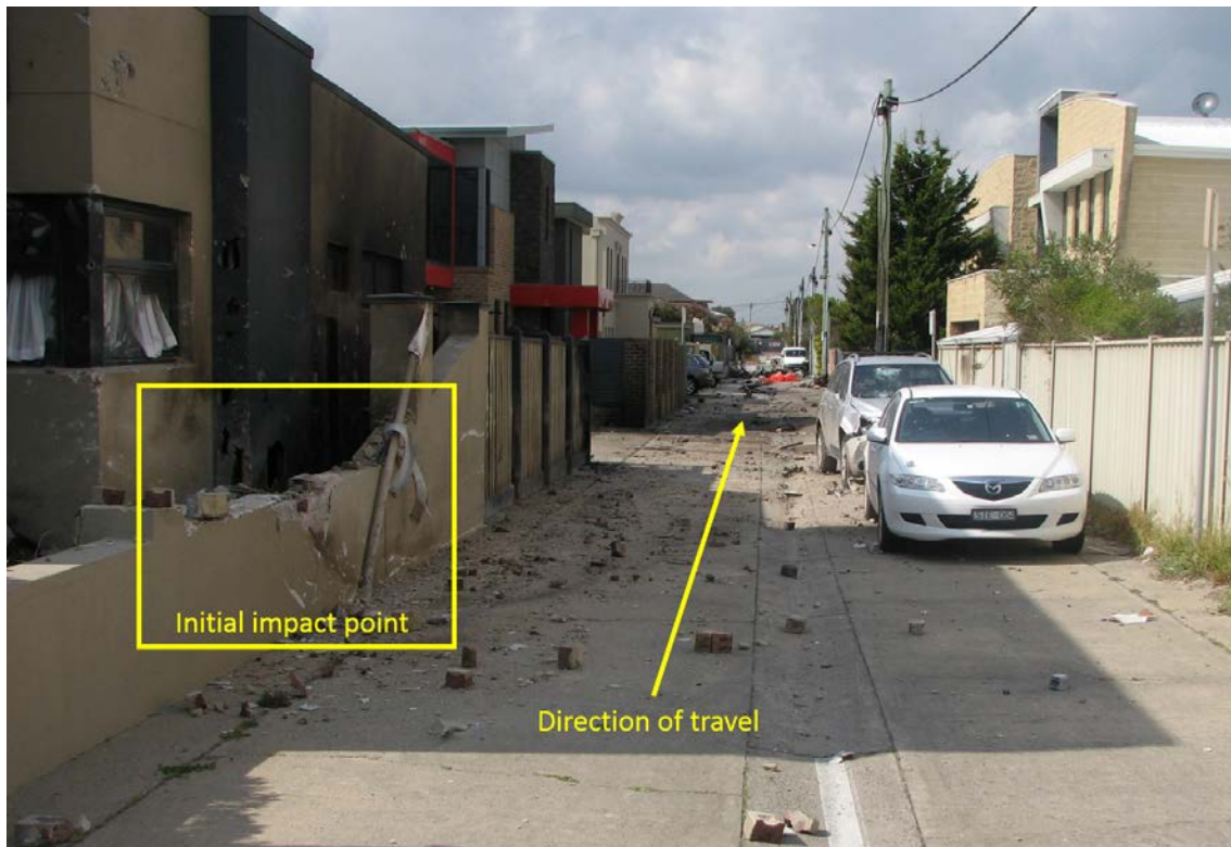
Figure 1: Accident site from the initial impact point on the left, looking south down the laneway
