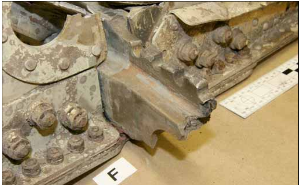
Figure 8. Underside of right wing attachment lug showing tearing along flange section
