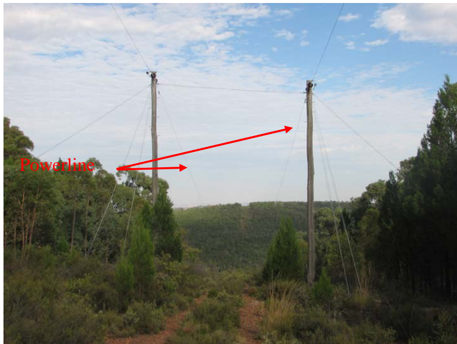
Figure 4: View of the eastern power poles, looking west
