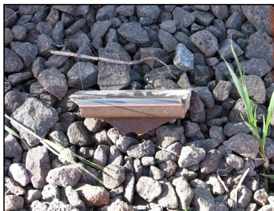
Figure 4: The ejected rail piece in-situ
