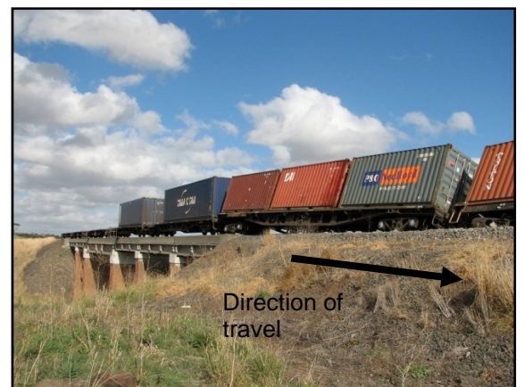
Figure 1: Point of derailment on bridge
